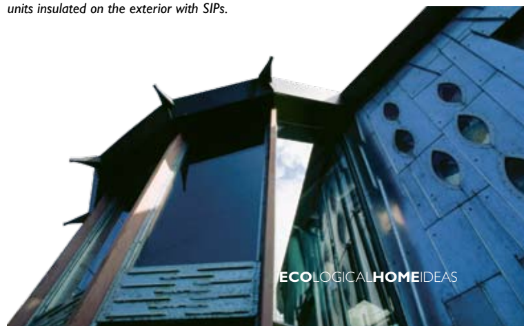
The walls are 6-inch-thick concrete masonry units insulated on the exterior with SIPs.
